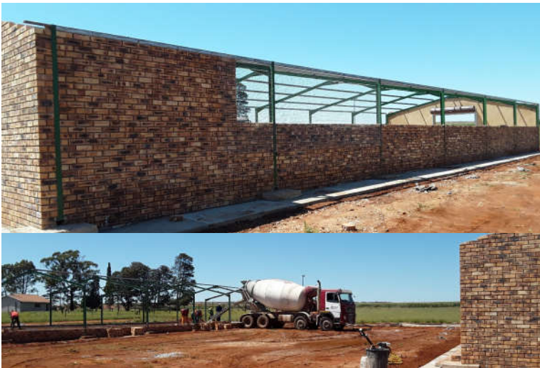
Poultry Construction Project
